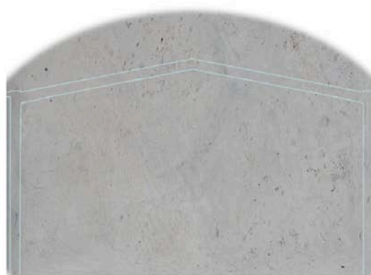
TRACE 1ST PORTAL FRAME TO USE AS A TEMPLATE FOR OTHER FRAMES
